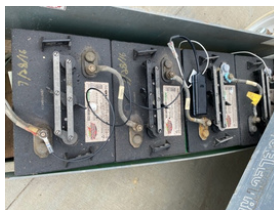
Power source located on a scissorlift.
